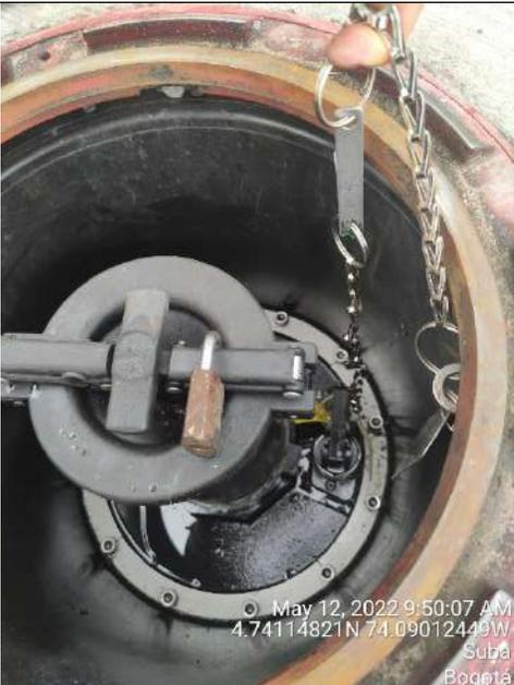
Foto 14. Spill-container gasolina corriente- tanque 1
