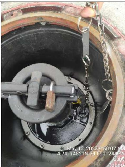
Foto 14. Spill-container gasolina corriente- tanque 1
